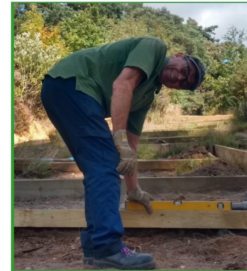
Step repairs on Oxshott Heath
