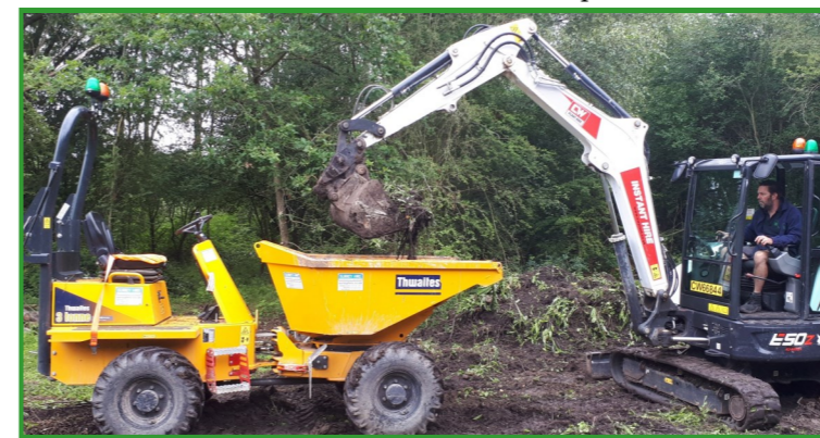
Excavating new pond at Hollymoor Grove, HCP
